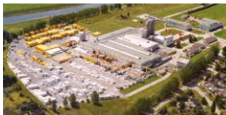
Calbe Factory, Germany
