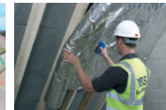
YBS SuperQuilt being installed under rafter
