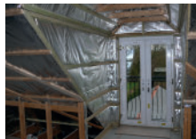
YBS SuperQuilt being installed in a dormer
