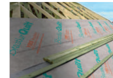
YBS BreatherQuilt being installed over rafter
